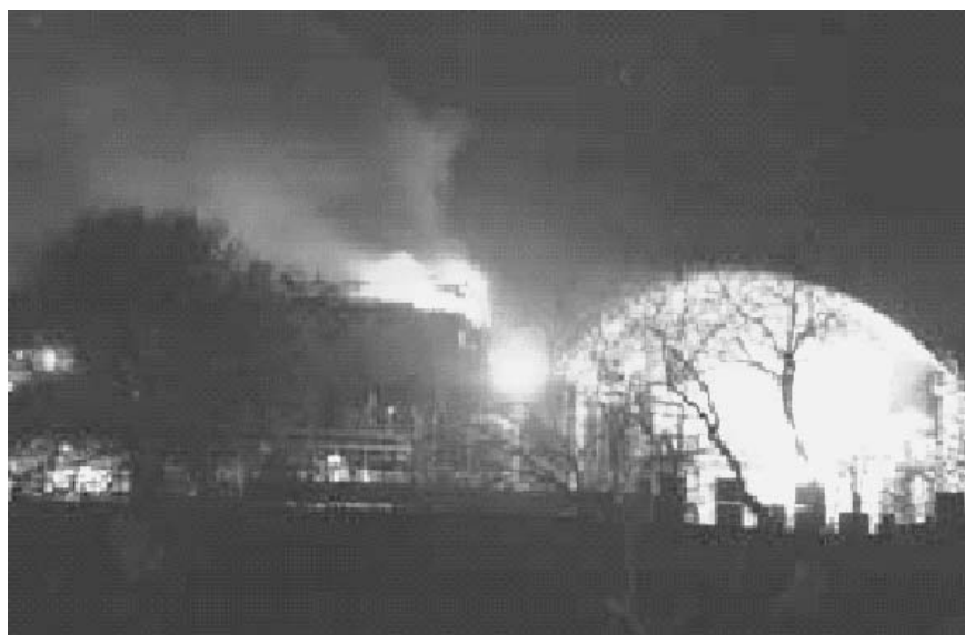
Morton International Inc after the explosion and fire, caused due to a runaway reaction that released flammable materials
